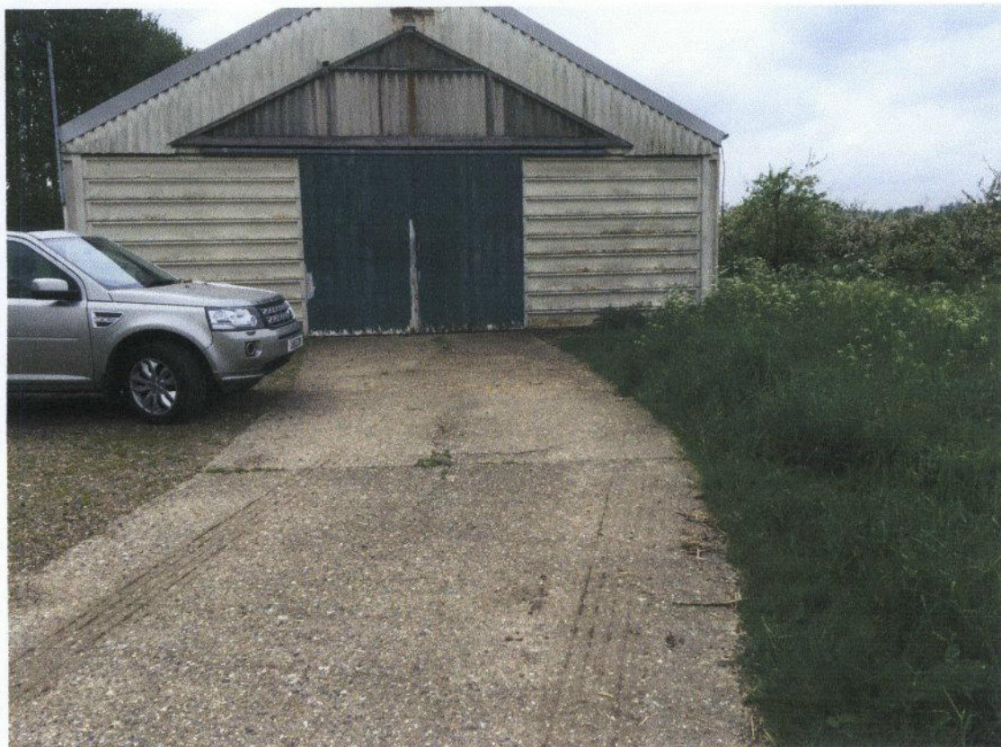
Exterior showing parking and level access to building
